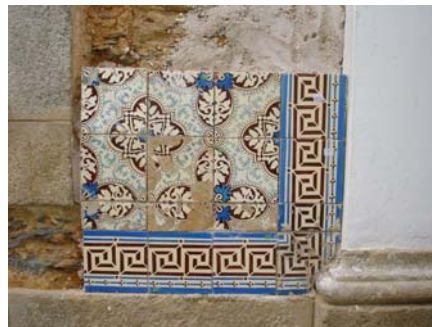
Fig. 68 - Painel com argamassa CRM
