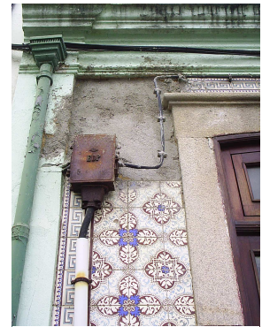
Fig. 2 – PRU 1, showing a gap of tiles.
