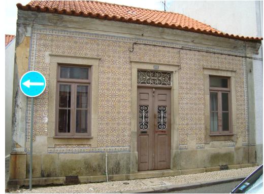
Fig. 1 – PRU 9, before intervention in the PRU program.
